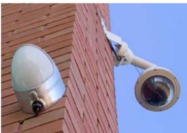
CCTV can be used to aid the security of a site and can act as a deterrent to criminal activity. It is important that the intended use of the CCTV system is known at the planning stage as this will affect the type, quality and quantity of equipment required. The availability of power to the CCTV system and lighting should be considered. Many different types of equipment are available with low light or infrared operation or combined with white or infrared lighting units.
