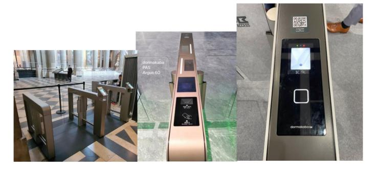
Care must be taken to ensure the access control reader choice is compatible with the usage and speed of the chosen turnstile. Proximity readers will provide a higher flow of traffic, whilst bio-metric readers may cause slow passage through the chosen turnstile.
